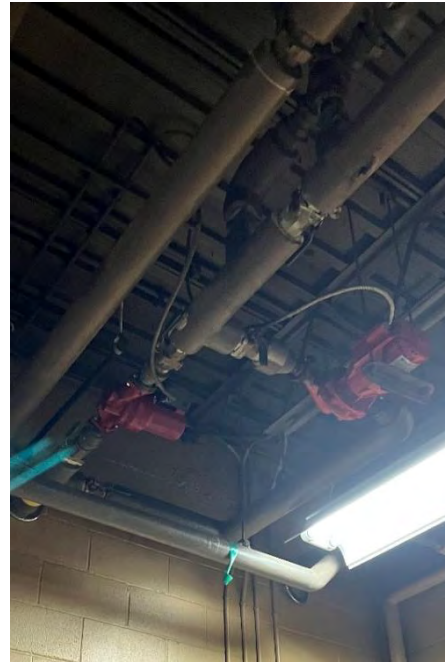
Figure 10 Hot water recirculation loop
