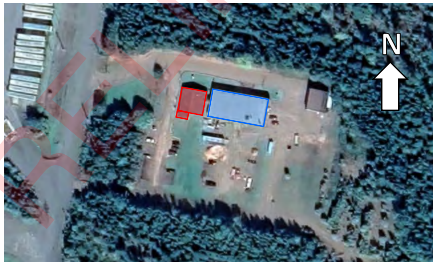
Figure 1 – Plan view location and orientation of Building A (shaded red) and Building B (shaded blue) of the Colchester Water Utility Administration facility, Debert (Google, 2022)
