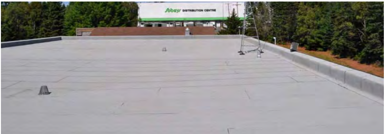
Figure 1 Roof drains over service area of building
